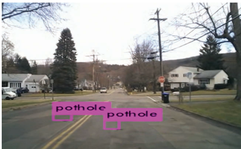
FIG4 Potholes can be detected with deep learning.
